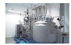
Distilled water system to ensure endotoxin below 0.015 EU/ml
